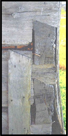
Typical southern Illinois log house, half-dovetail corner notch.
