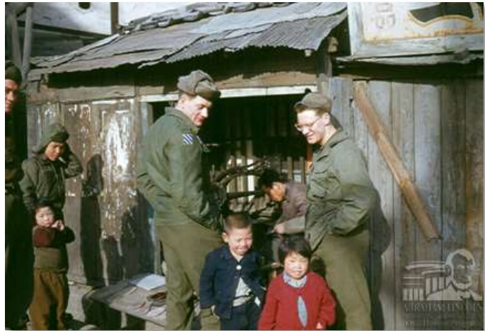
Early in 1954, while attending a library school in Seoul, Maras snapped a photo of two buddies, while they visited a neighborhood in Seoul. South Korea was devastated by the war, so Koreans used whatever building materials they could find.
