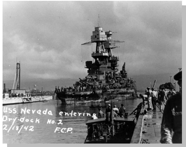
*Tripod masts replaced the USS Nevada’s cage (or lattice) masts, the type of observation masts that were common on major warships in the early 20th century.*
