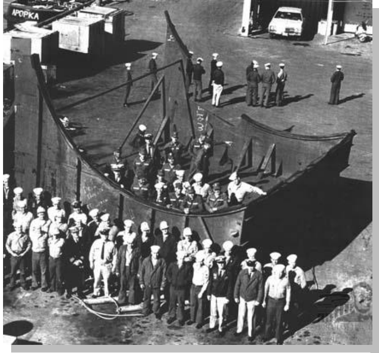
This cofferdam was built for SSN George C. Marshall on the pier where the USS Canopus AS-34 docked in Rota, Spain in 1967. The Marshall had been rammed by a Russian trawler (spy ship).
