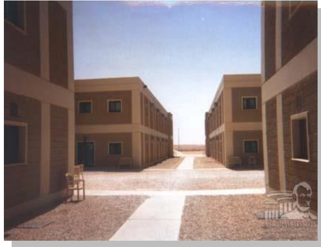
The Civil Engineering section billeting area in the cantonment area at the Prince Sultan Air Base in Saudi Arabia in February, 2000.
