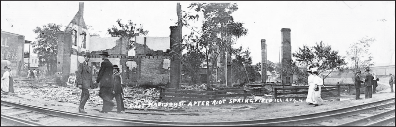
Sunday strollers view burned homes on East Madison Street (top) and at Twelfth and Mason streets (bottom).
